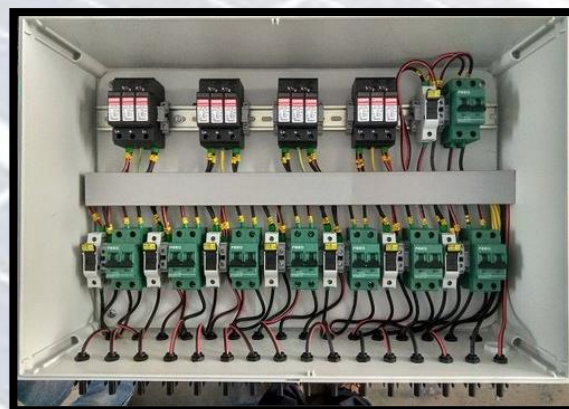
DCDB IP65 PC Enclosure with MC4 Connectors
