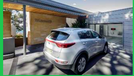
A flexible and cost-effective battery storage solution for a high-end residential development
